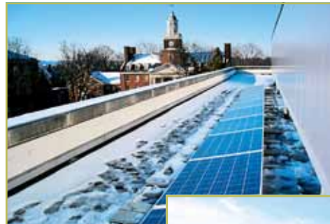
Images top to bottom: Photovoltaic panels, Acopian; Photovoltaic array, Metzgar; Vegetated roof, Acopian.
